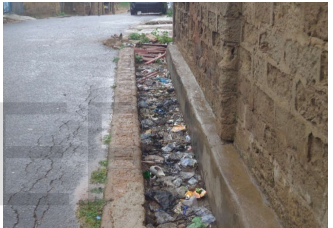
Plate 8. Refuse found inside an existing Drainage in Kube-Atenda
