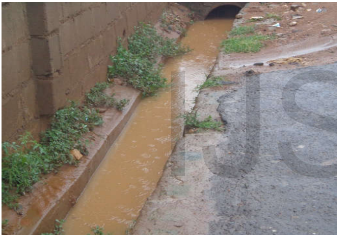
Plate 1. Section of a Road in Kube-Atenda showing blocked Drainage/Culvert
