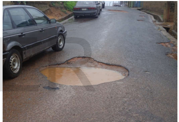
Plate 2. Pot Hole - a devastating effect of flood on a tarred road in Kube-Atenda
